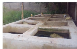
Testing stage of the pond
