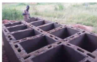
Construction of Pond
