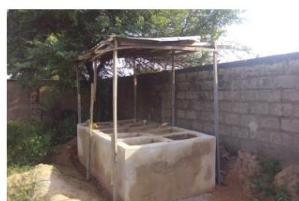
Testing stage of the pond
